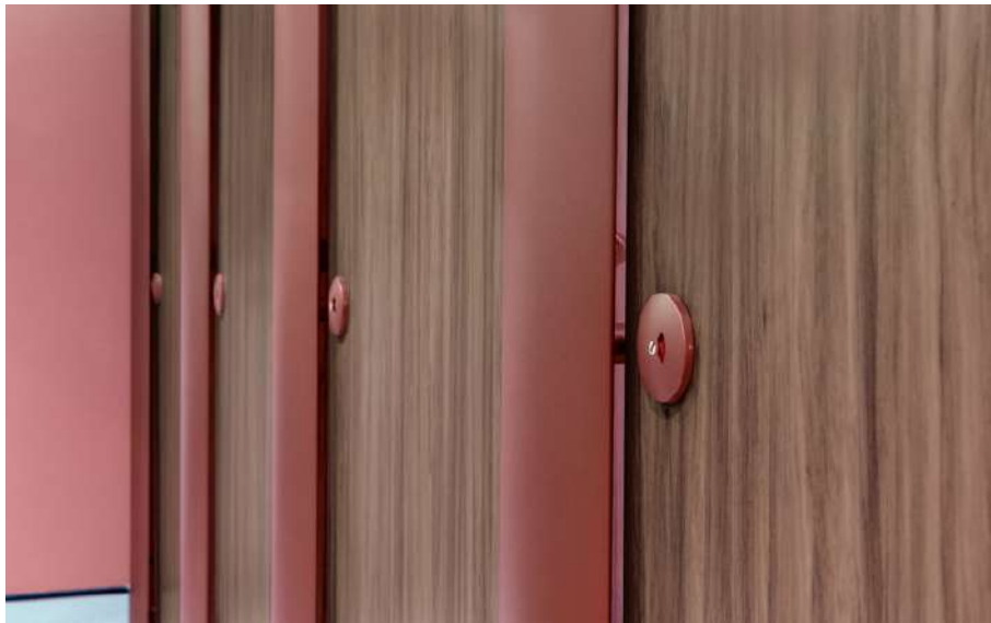
Curved aluminum pilasters
