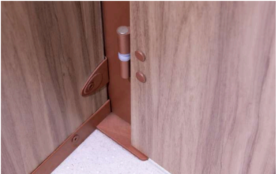
Bolt through brackets and hinges
